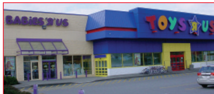
The Side By Side concept began in Canada in 2002. The third store to be expanded in that format was #3533 Coquitlam BC.
